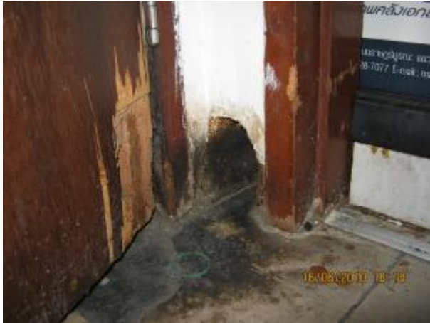
At the Edge of the door , rodents make the damage as the way to go in and out
