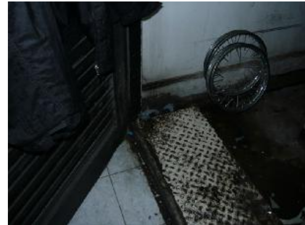
At the door corner , rodents use the hole for way in and out
