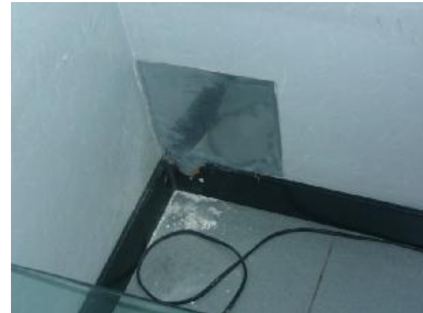
We use metal sheet to close the hole to protect rodents run in the facility
