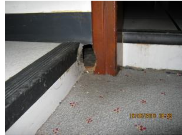
At the Edge of the door , rodents make the damage as the way to go in and out
