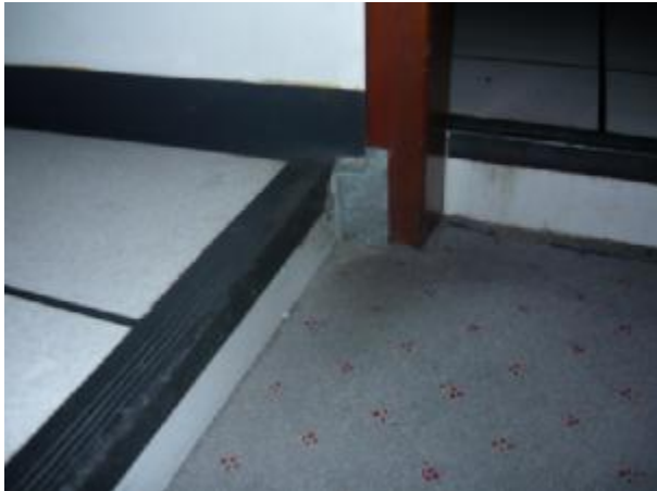
We use metal sheet to close the hole to protect rodents run in the facility
