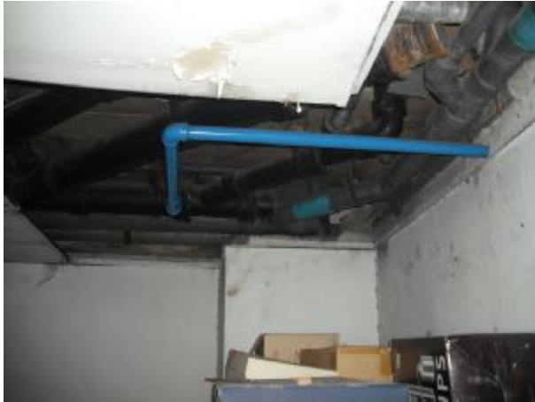
rodents can use the pipe line as the way to run in and out of the customer facility
