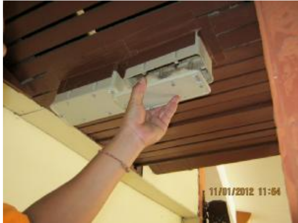
In case we found too much termite , we will put 2 stations together
