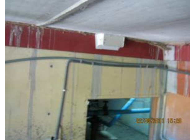
After finish on ground termite bait station
