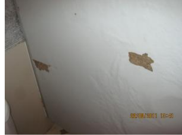
Termite attack the built in furniture
