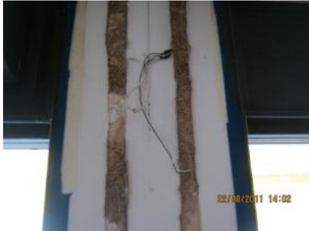
Structure of the wood has been destroyed by termite
